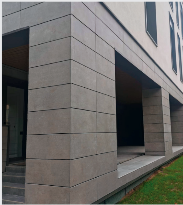
Spain, Pamplona Residential building
