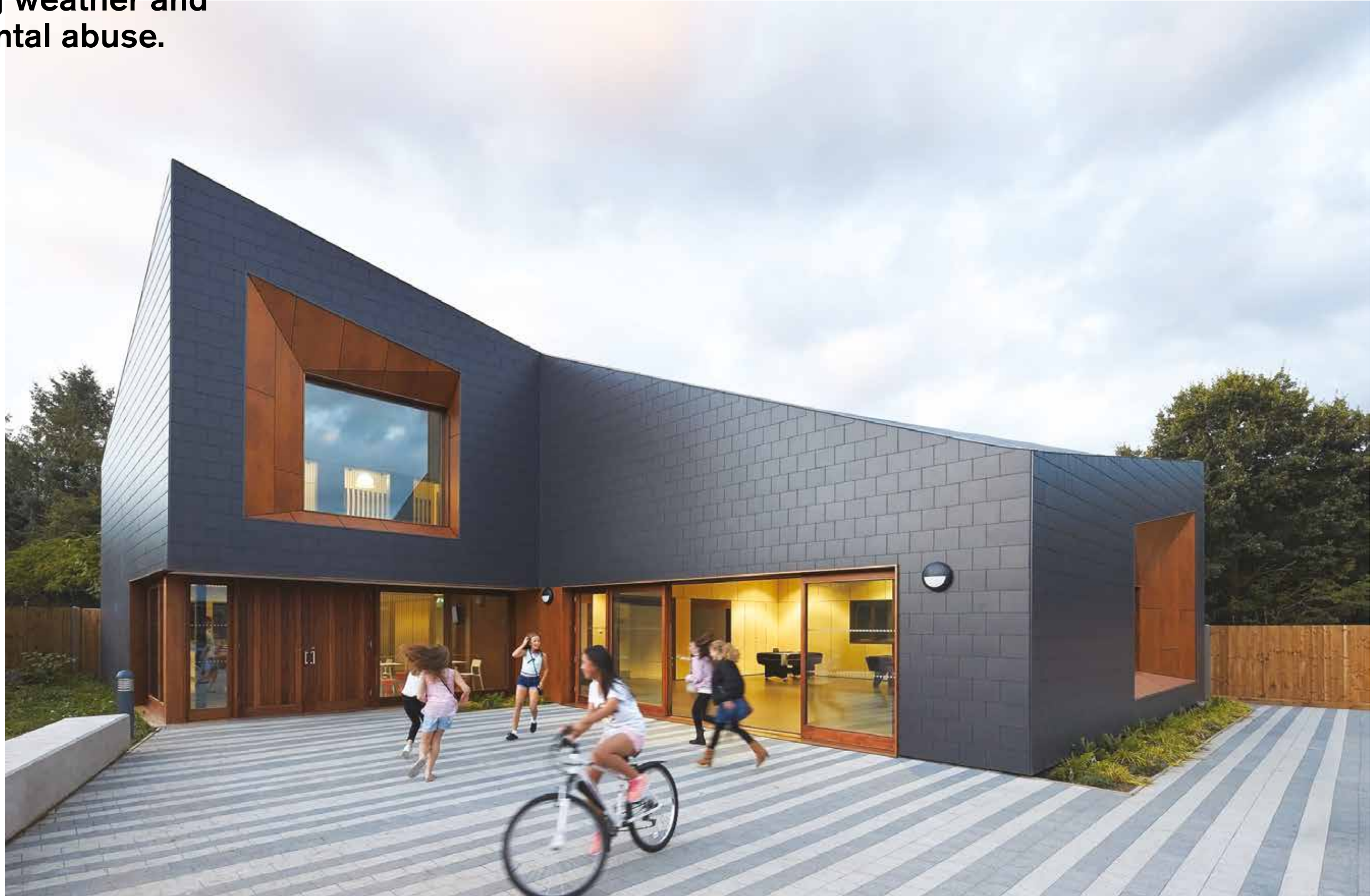
Facade Exterior cladding
