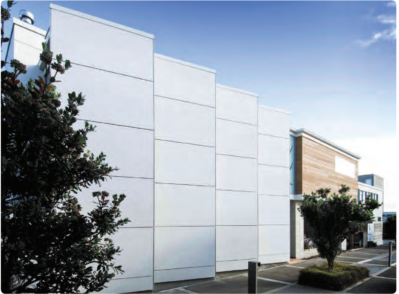
RESIDENTIAL BUILDING, NEW ZEALAND (PHOTO EURO PANELS)
