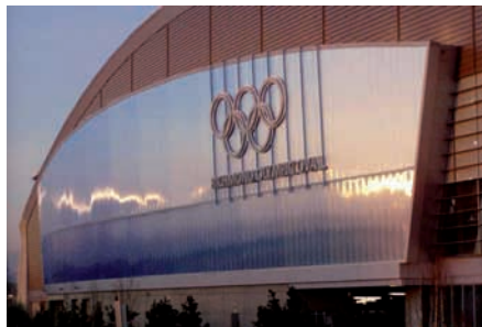
An adjacent light source creates a "bolt of lightning" shimmering across the entire façade.
